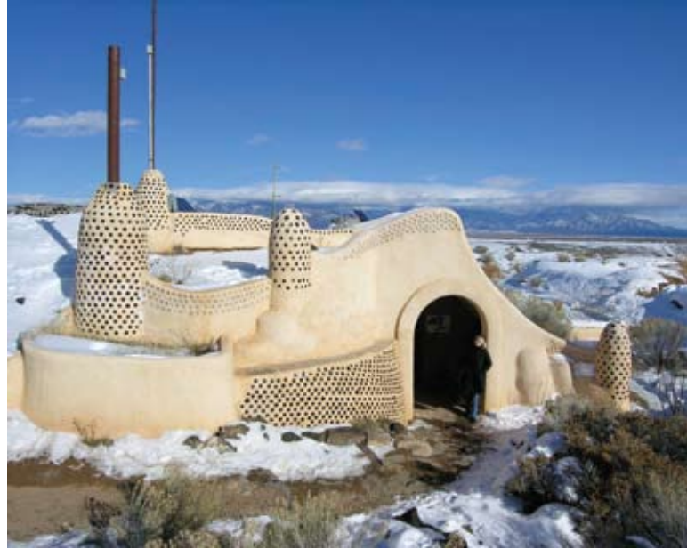
In the Earthship Community, a group of passive solar homes made of natural and recycled materials outside Taos, New Mexico, the cycle of the ever-changing seasons is always readily apparent.
